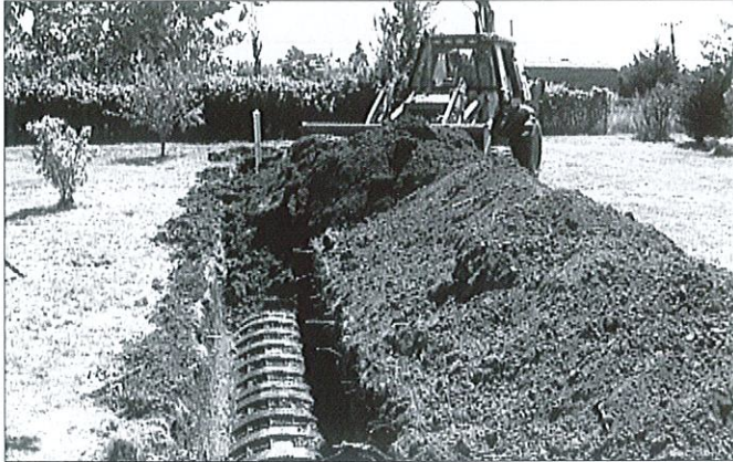
Backfill the trenches.
