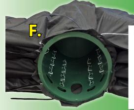
F. Overlap remaining fabric to cover the FDU Connect Zip-Ties to Upper and Lower Zip-Tie Grooves to secure Treatment Fins to FDU
